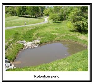
Flood control reservoirs are most commonly built for one of two purposes. Large reservoirs are constructed to protect property from existing flood problems. Smaller reservoirs, or detention basins, are built to protect property from the stormwater runoff impacts of new development.
